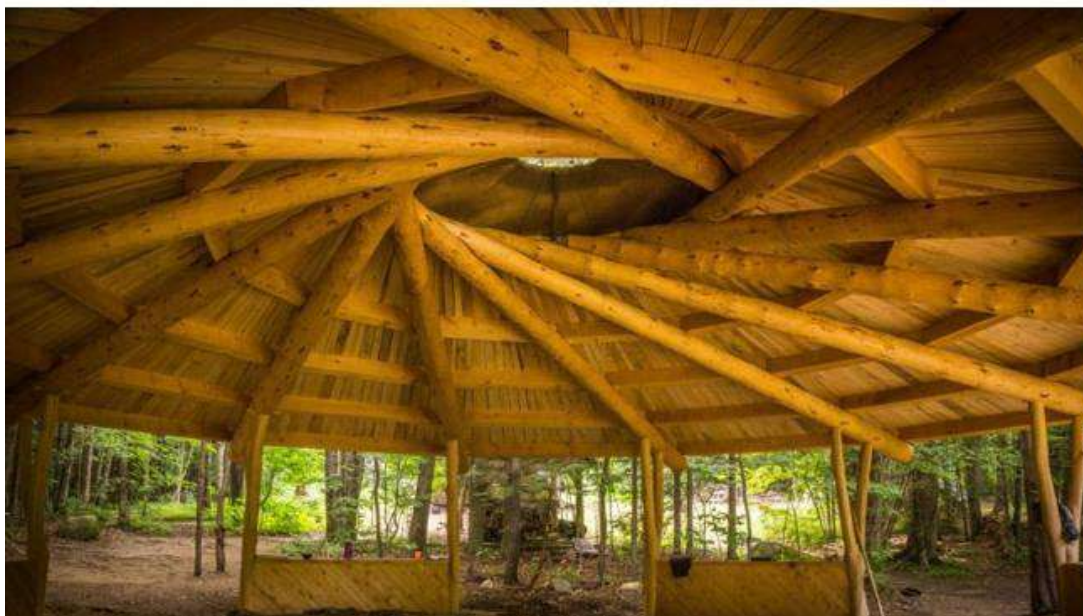
Design proposal for a reciprocal roof at the woodland hub in Rhondda Cynon Taff
